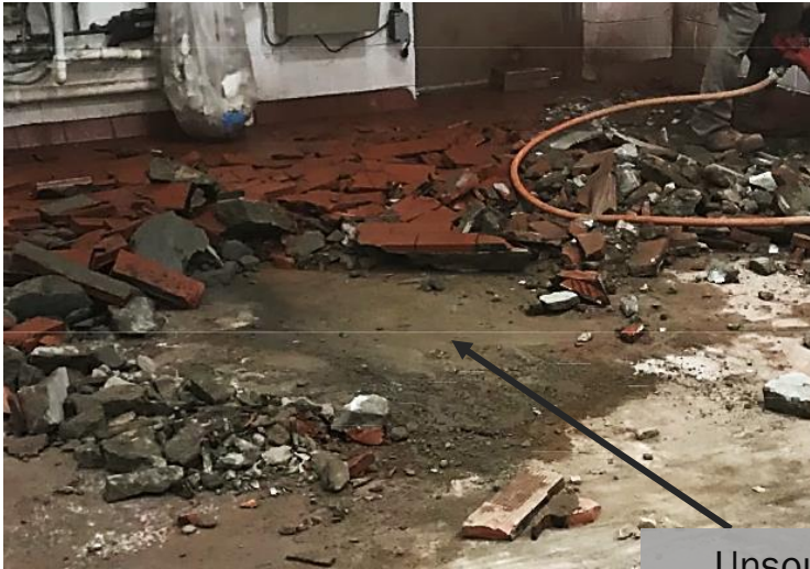
Unsound Brick and Contaminated Grout Bed
