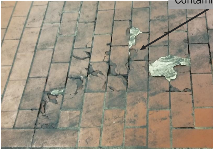
Unsound Brick and Contaminated Grout Bed
